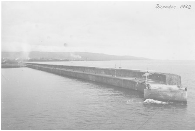
Figure 4. Photograph of the outer breakwater of the Port of Catania captured after the completion of its 200 m-long extension. The image shows the triangular service area located at the junction between the original outer breakwater and its extended section (source: F. Pesce, 1932).
