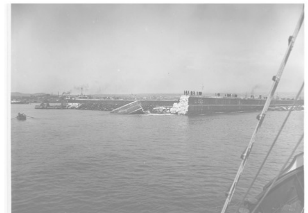
Figure 6. Photographs taken on March 31st, 1933, a few days after the sea storm that caused the destruction of a section of the outer breakwater of the Port of Catania, extending from the triangular service area to the head (source: F. Pesce, 1933).
