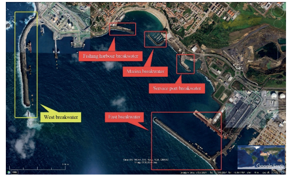
Figure 2. Rubble-mound breakwaters at the port of Sines
