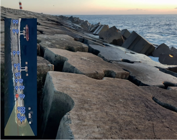
Figure 6. 2018 visual observation at point 27F (F – front direction) of the Sines west breakwater (outer armour layer)
