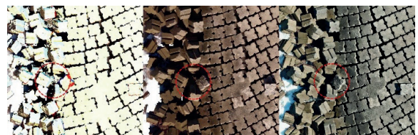
Figure 20. West breakwater. Changes detected between 2020 and 2022 – Occurrence 3 – Section G
