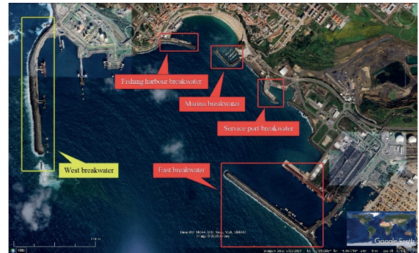
Figure 2. Rubble-mound breakwaters at the port of Sines
