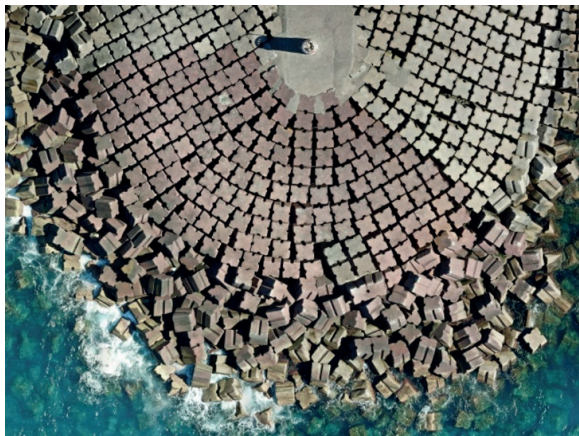
Figure 17. Detail of the orthomosaic of the Sines west breakwater (head section)
